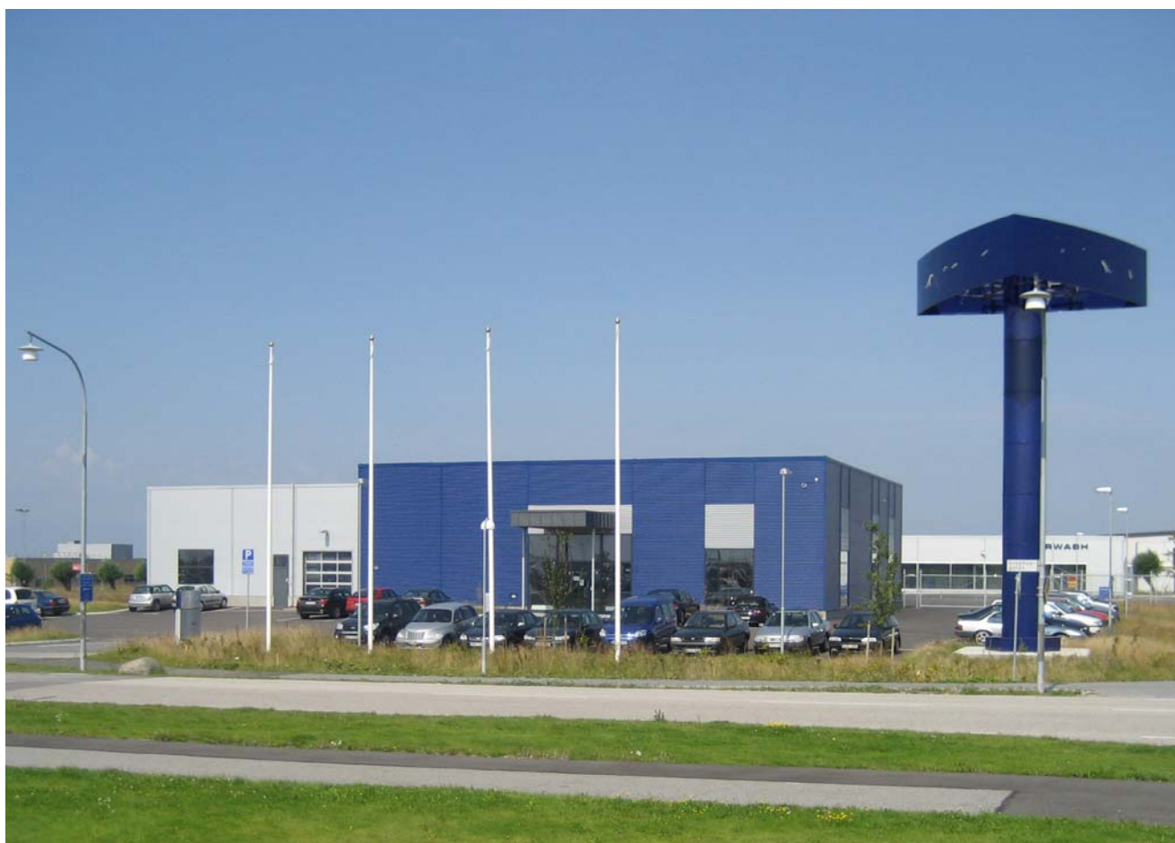
Malmö Urnes 1, Svågertorp (The property was acquired in June 2007.)
